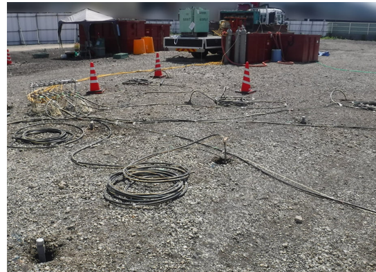
In situ bioremediation* site where SoyBio MA is delivered via a well
