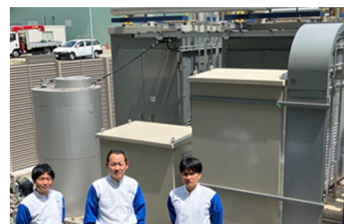
Biomass boiler at Fuji Oil Co., Ltd. Chiba Plant
