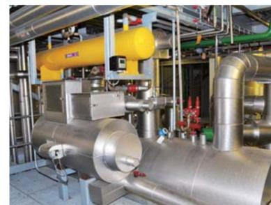
Ice condenser-type vacuum generating apparatus
